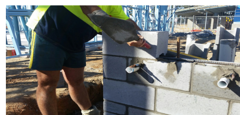
INSTALLATION OF A MASONRY WALL WHERE THE WATER BUBBLERS FOR A JUNIOR GLA RESIDE
