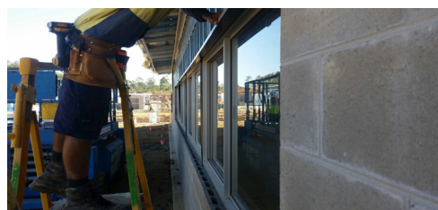
INSTALLATION OF THE SECONDARY HEAD FLASHING ABOVE WINDOWS TO THE SOUTH ELEVATION OF THE RESOURCE CENTRE
