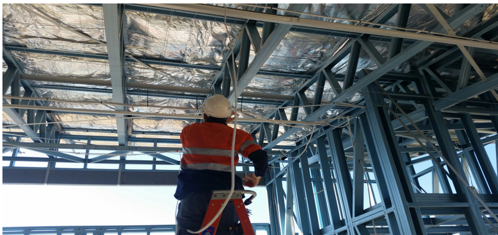
INSTALLATION OF ELECTRICAL CABLING IN THE CEILING OF A PREP LEARNING GLA
