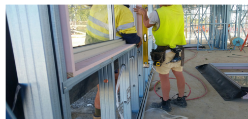
INSTALLATION OF A SLIDING WINDOW IN THE GLA OF A PREP LEARNING CENTRE
